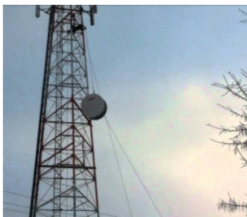
Removing a 6' microwave dish. Image via YouTube
